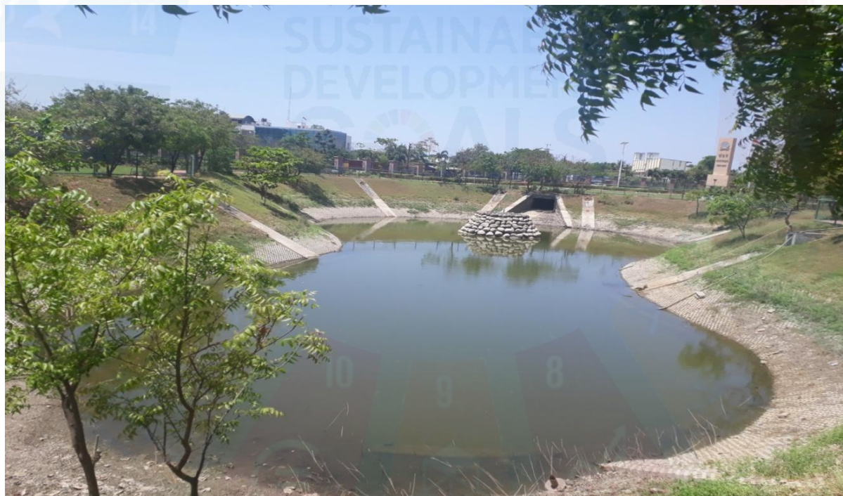
Rain Water harvesting pond
