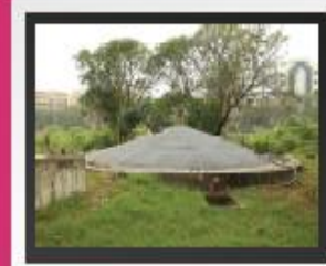
BIO GAS PLANT
